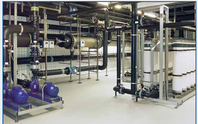
Fig. 11 drinking and process water filtration in brewery
