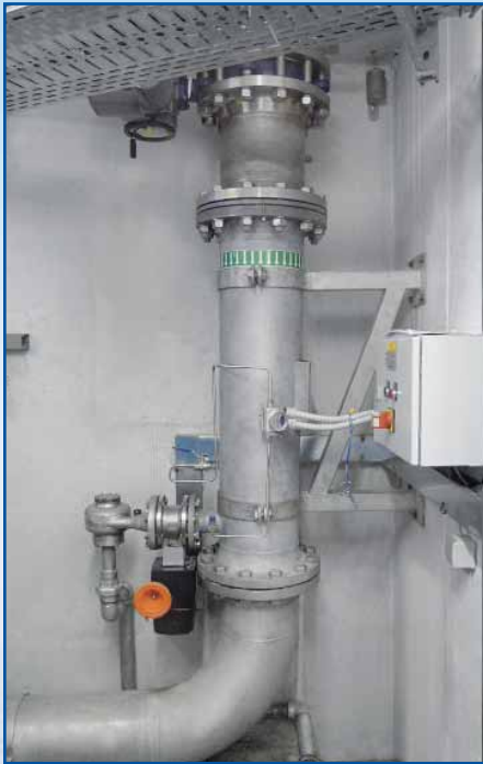
Fig. 8 sea water filtration for snow making system
