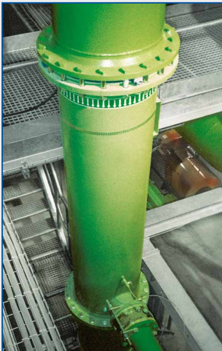
Fig. 10 cooling water filtration for CERN, Genf (European Organization for Nuclear Research)
